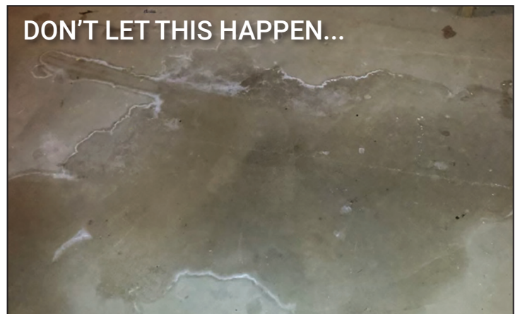
Without PolyCove, moisture can wick through the concrete and condensation puddles will form on the new floor.
