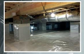
Fiber Reinforced Flexible Membrane
